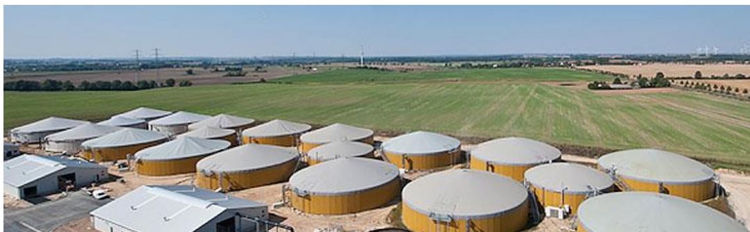
Figure 7: Biogas park Gustrow; The largest upgrading plant in Germany
