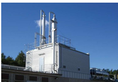
Figure 12: Chemical Scrubbing (Purac CAPure)
