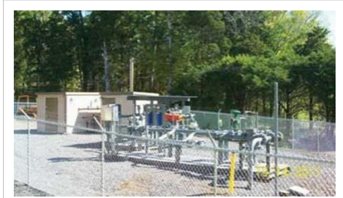
Figure 17: Upgraded landfill gas from Meadow Branch Landfill in McMinn County, Tennessee, is piped to Spectra Energy's East Tennessee Natural Gas
