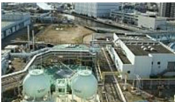
Figure 11: The Kobe Biogas Station for production and upgrading of biogas (from Sewage)
